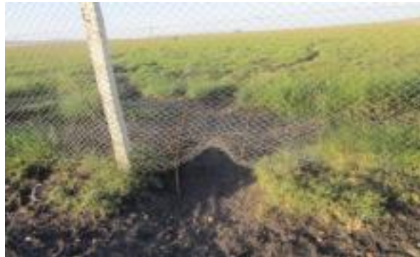
Figure 2: A part of Konza Technology City's perimeter fence, vandalised to graze cattle.
